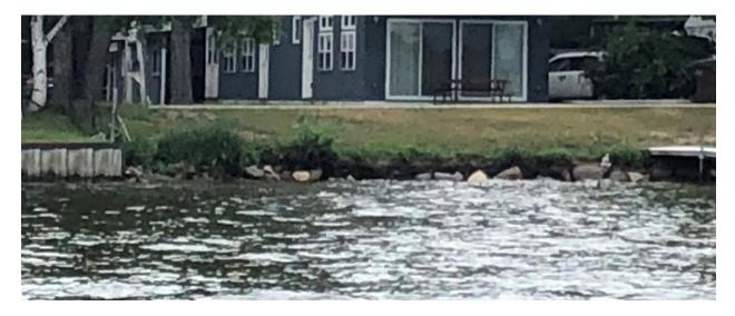
Figure 28. Rip-rap failure due to wave action and high-water levels.
